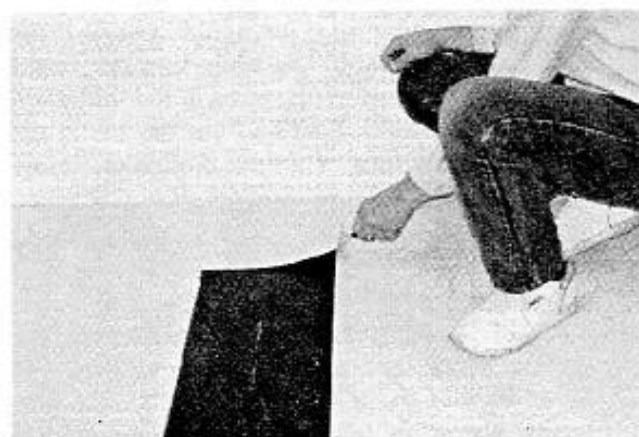
Removal of tile over subfloor joint.
