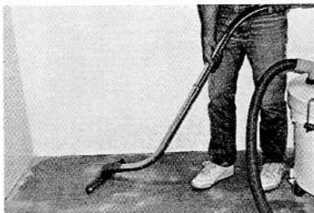
Vacuuming entire floor.
