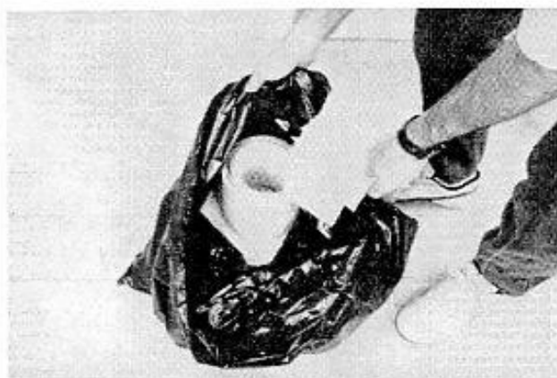
Placing felt scrapings and flooring strips in bag.
